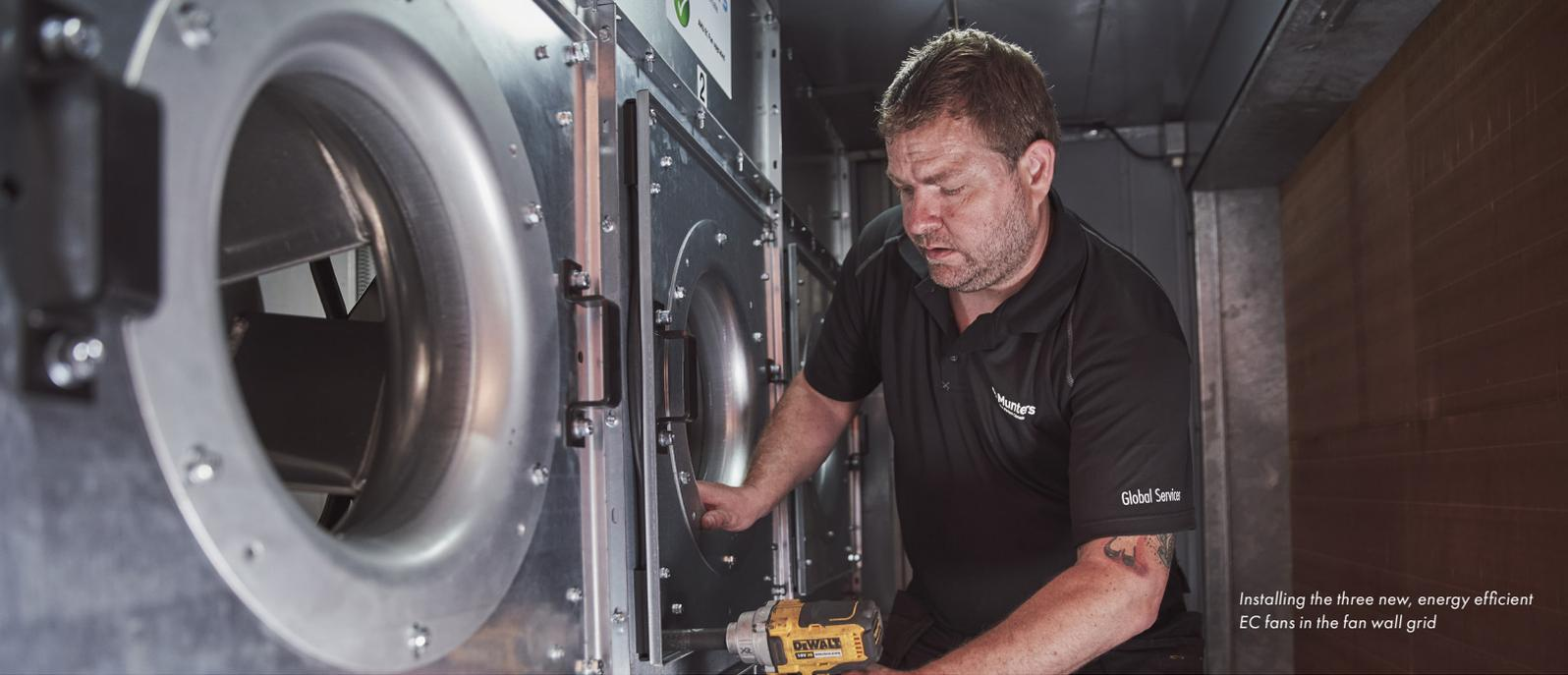
*Installing the three new, energy efficient EC fans in the fan wall grid*
